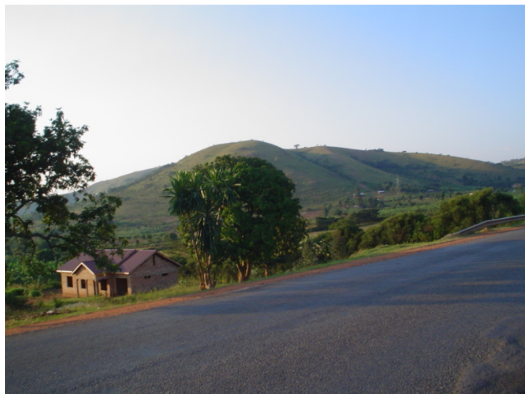
Figure 38. Part of a highway road within the Lake Victoria/Kagera Basin .
